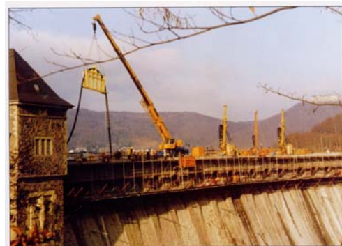
pic. 4.: installation of anchor
